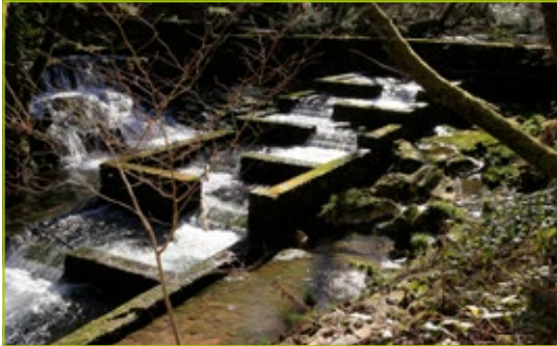
Fish ladder at the San Bartolomé hydroelectric power plant (Galicia, Spain).
