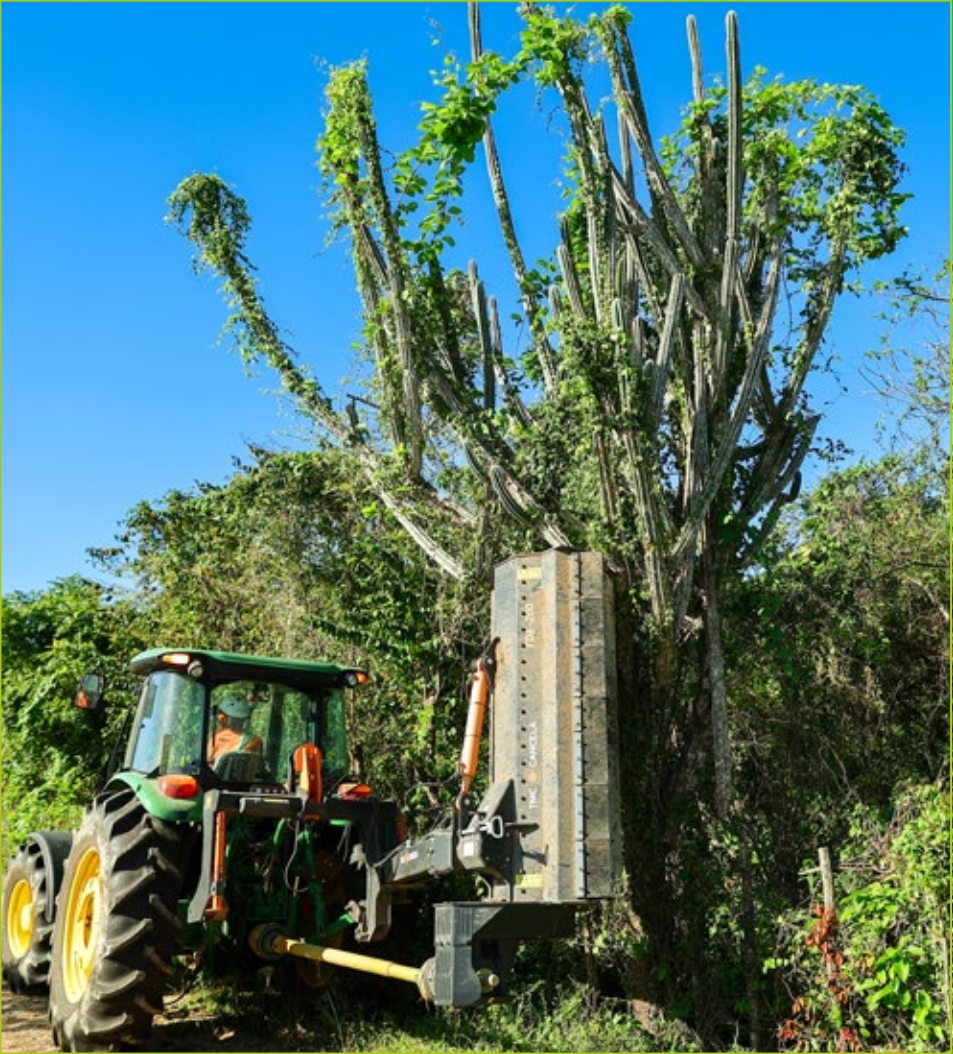
Enclosure of pitahaya in Cumayasa 1 and 2
