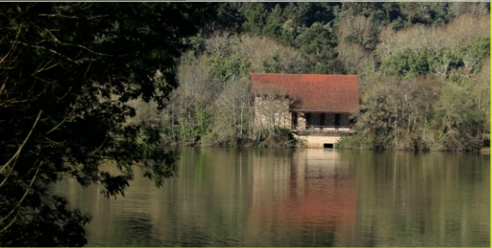
Ciervos hydroelectric power plant (Galicia, Spain).
